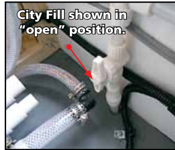
After hook-up, turn City Fill shut-off valve to "open".
