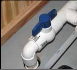
— OPEN — To Drain Tank
