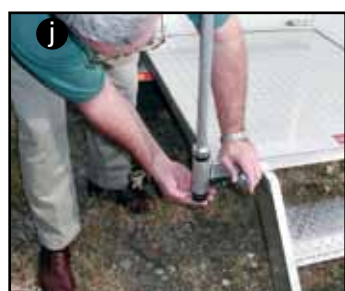
Secure railing by screwing in cap as shown.
