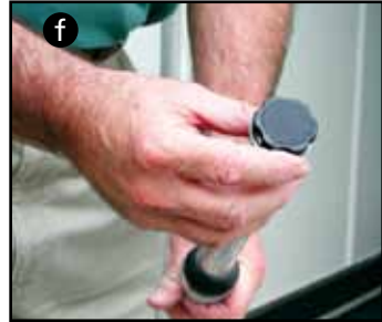
Unscrew cap from railing tube.
