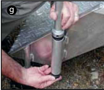
Insert railing tube, fasten with cap.
