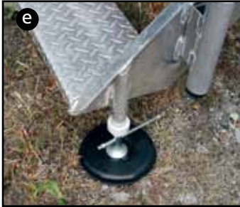
Place sand pad under step legs.
